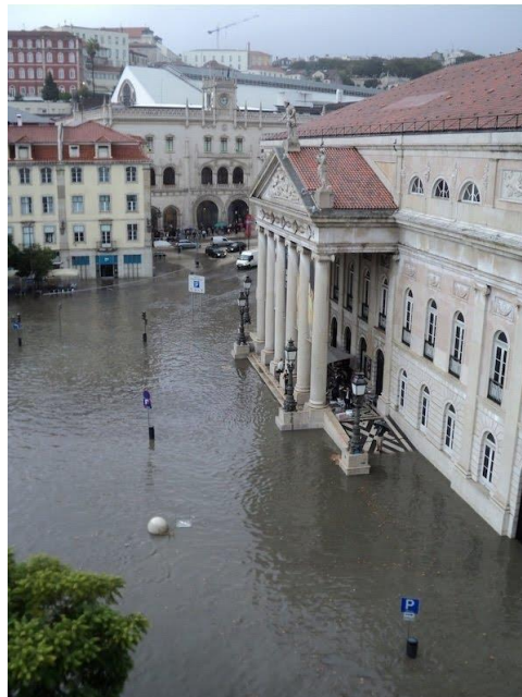
Figure 26: Inundation during the 2008 event (Front of the Theater)
